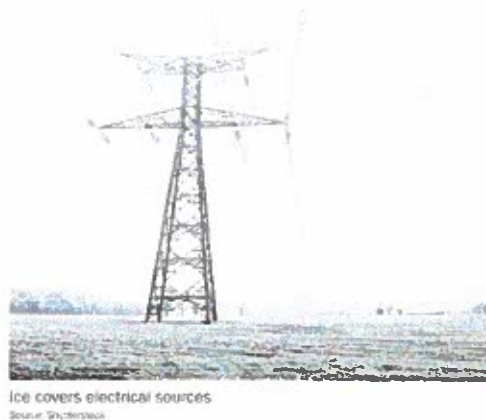
Figure 2: Nebraska and Kansas Electrical System Ice and Wind Storm Mitigation Projects hardened power lines against high winds and winter storm loads
