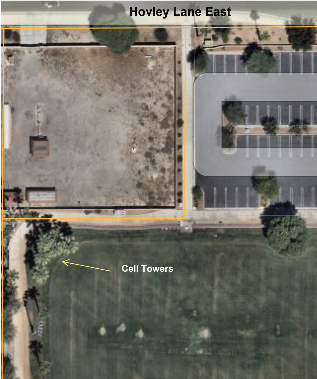
Hovley Soccer Park Cell Tower
