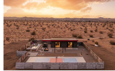
▲ A sport court is located within the building pad boundaries. See Standard 2.2.15.
