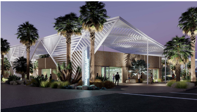
Simplifying and separating the structural system from shade canopies to reduce steel tonnage and foundation costs.
