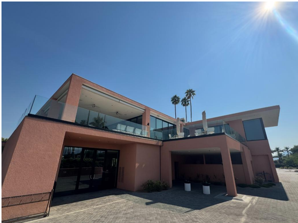
Figure 6 – Rear second-story terrace addition to clubhouse
