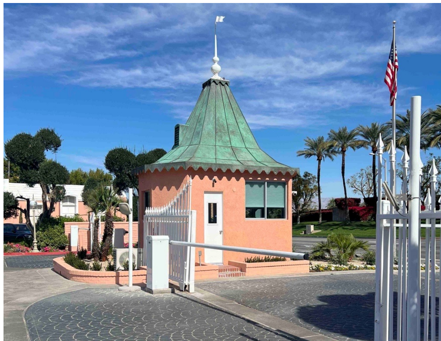
The south side of the structure is like the north side, with an inset window and single door. South elevation, view north.
