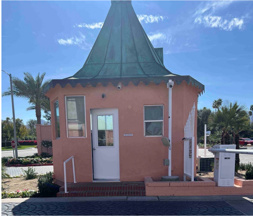
The copper roof wraps around the entire structure. On the north side is a single door and two windows. North elevation, view south.
