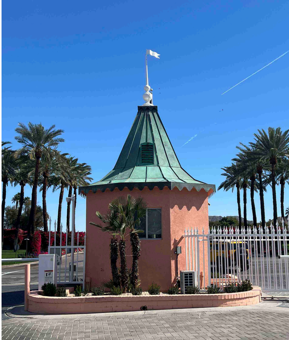
The rear of the gatehouse has a symmetrical footprint to the front elevation, with a single window placed in the center. The copper roof also features an inset vent. Rear elevation, view east.
