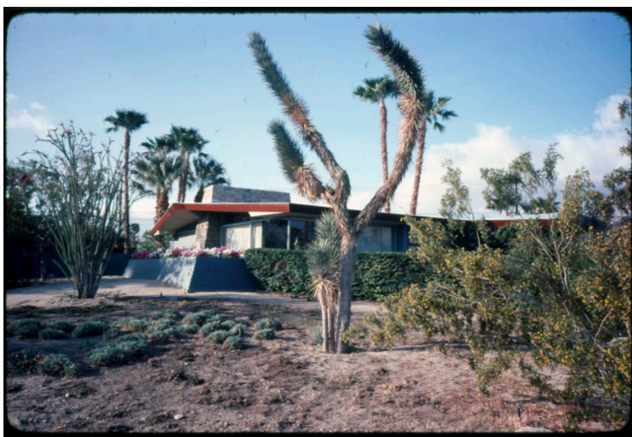
Figure 1.3. The Edgar W. Stewart house designed by Walter S. White in 1951, embodying the new direction of postwar "Desert Modernism." Photo courtesy of the Walter S. White Papers, Architecture and Design Collection, UCSB.
