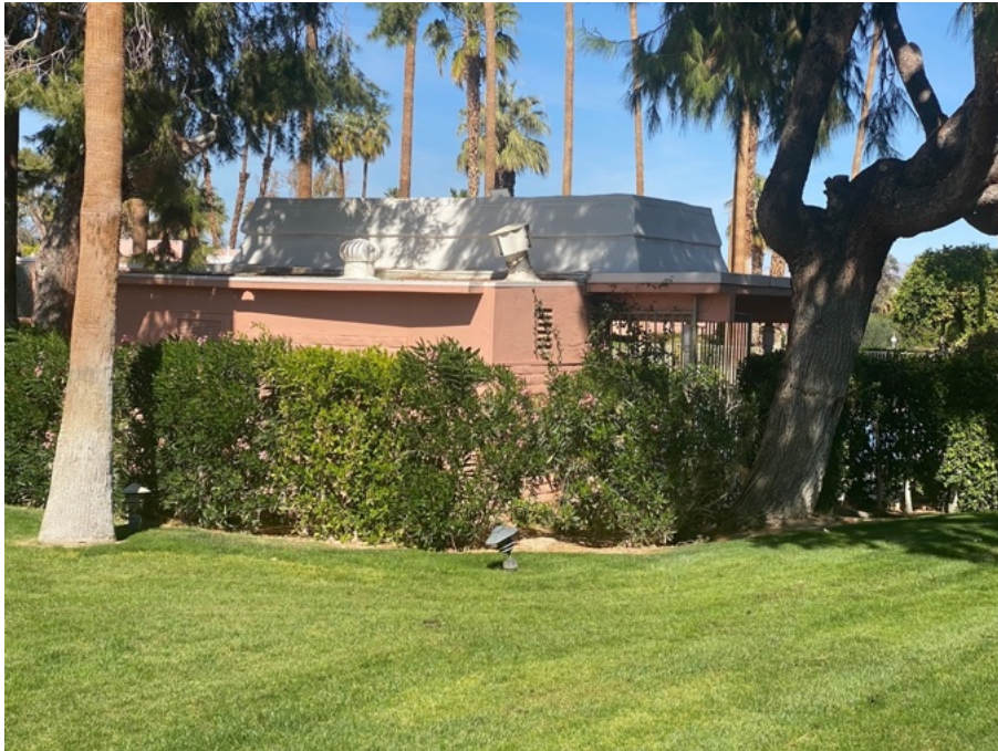
From the rear, the addition is a simple structure made of slump block and the mansard roof is visible.
