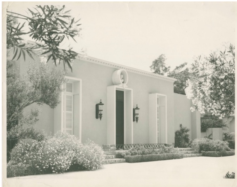
Figure 2.3. Woolf's Menefee house in Beverly Hills featuring tall volumes and historicist detailing. Photo courtesy the John Elgin Woolf Papers, Architecture and Design Collection, UCSB.
