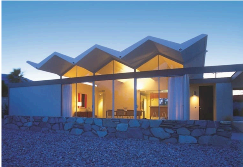
Figure 3.4. The iconic folded plate roof Steel Home designed by Wexler and Harrison in 1961-62. Photo reproduced from Palm Springs Life.
