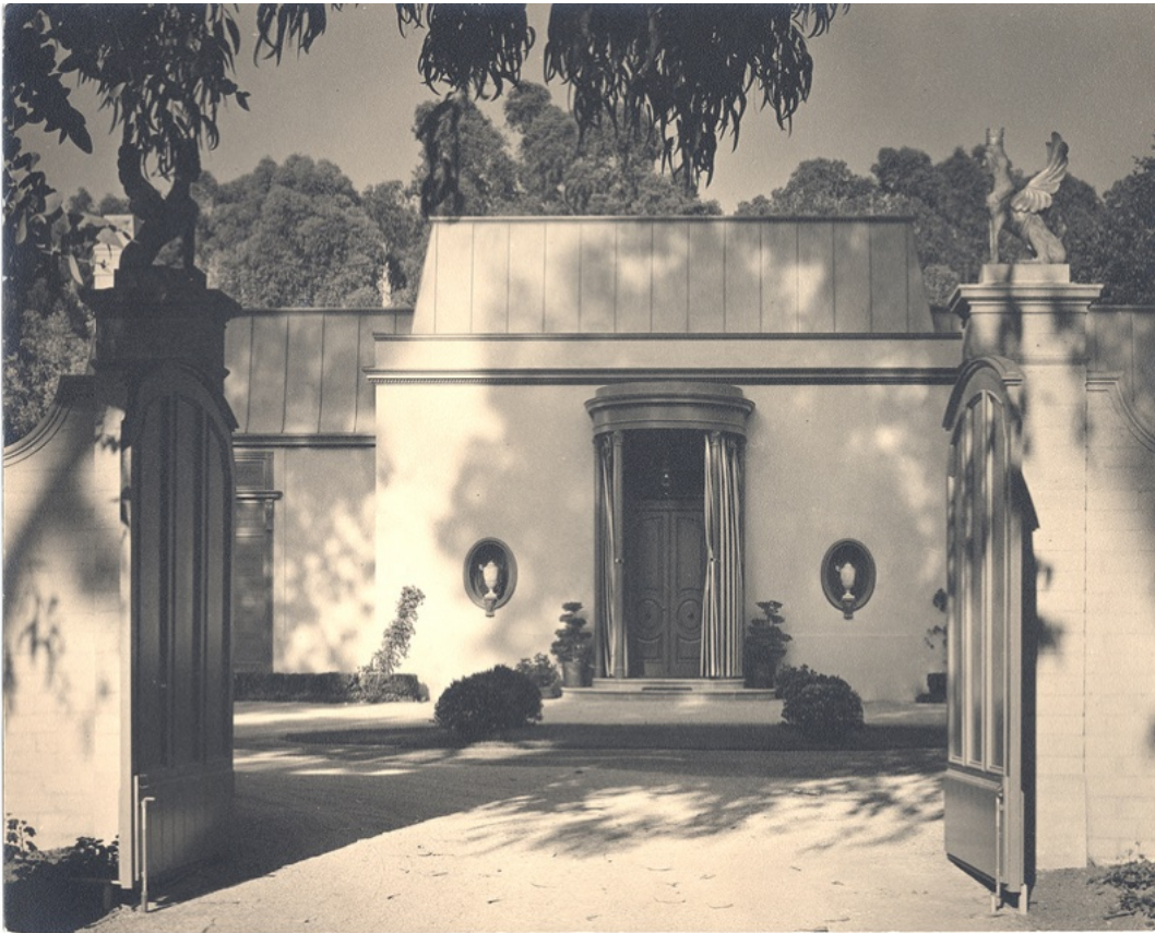
Figure 2.2. Woolf's seminal Pendleton estate (1942) in Beverly Hills with a landscape design by Tommy Tomson, later photographed by Slim Aarons. Photo courtesy the John Elgin Woolf Papers, Architecture and Design Collection, UCSB.
