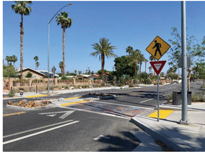
(A curb extension at a midblock crossing location. Source: Palm Desert Safe Routes for Older Adults Walk Audit)
