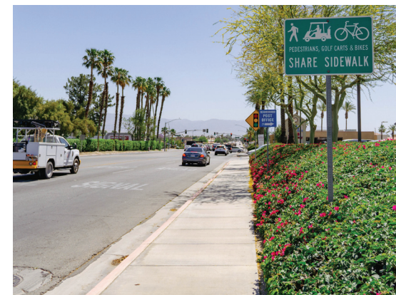
The shared sidewalk on the south side of Hovley Lane does not have enough space for users to comfortably pass each other.
