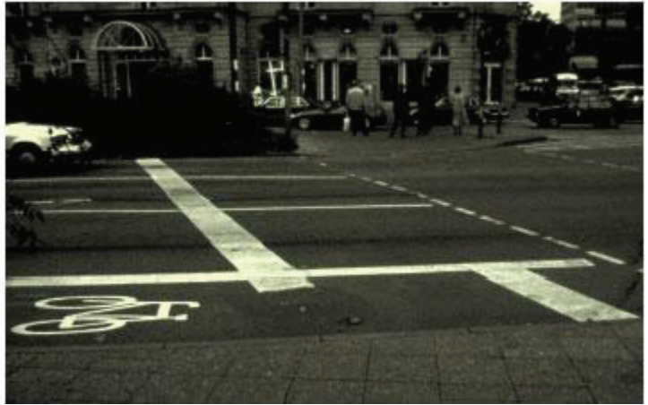
(Recessed stop lines are used at this signalized mid-block crossing to improve sight distances and to give the motorist who initially fails to see the crosswalk more time to stop. The cyclist can advance ahead which aids in cyclist safety, particularly with right-turning motorists. Source: FHWA.)
