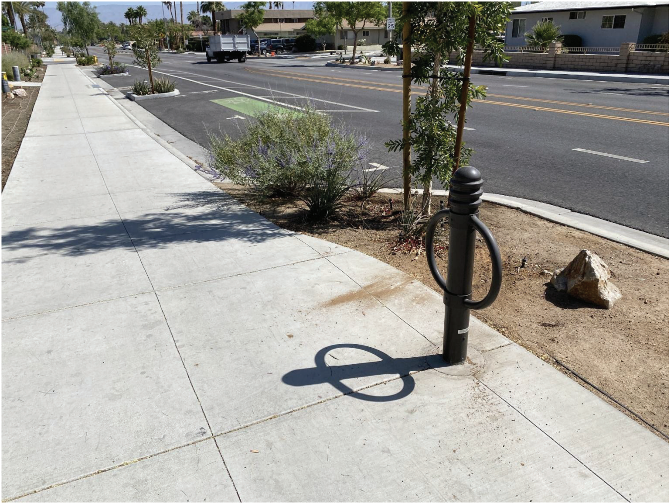
Figure 6. Bike rack and Class IIB Buffered Bike Lanes on San Pablo Avenue
