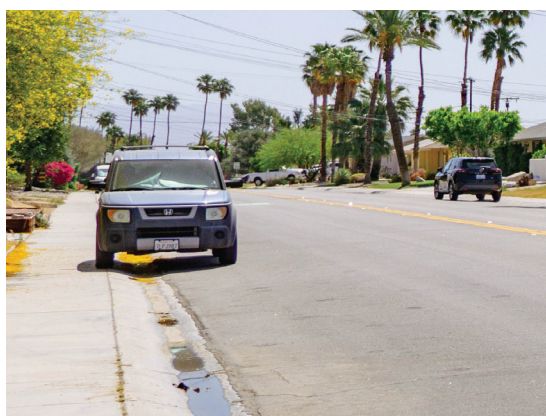
Rounded curbs lessen the division between spaces for pedestrians and cars in residential areas.
