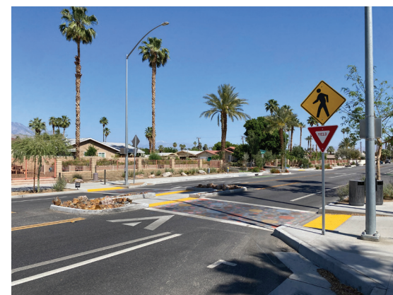
Creative and high visibility crosswalks, pedestrian islands, Class IIB buffered bike lanes, and pedestrian and bicycle amenities including benches, bike racks, and trash cans were recently installed along San Pablo Avenue.
