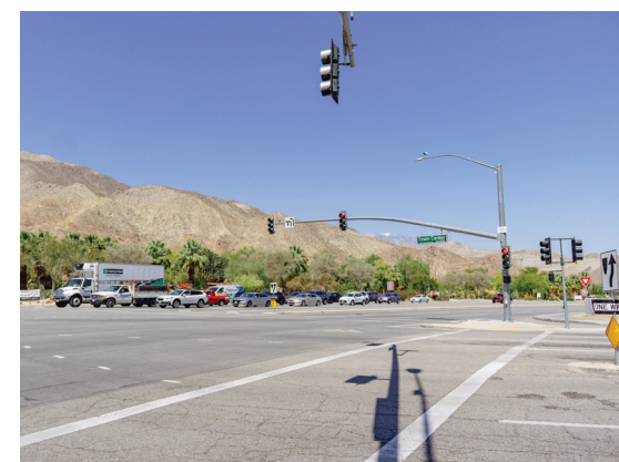
Participants stated it is difficult to see pedestrian signals at large intersections along Highway 111.
