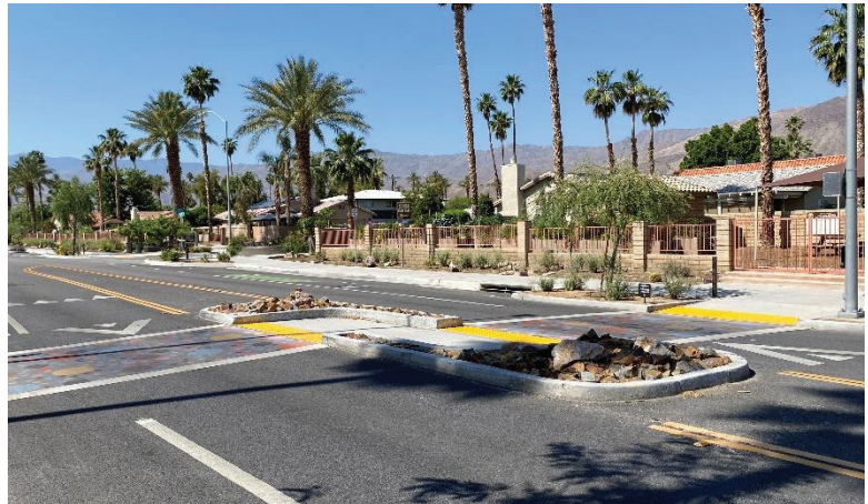
(A pedestrian refuge island at a midblock crossing location on San Pablo Avenue. Source: Palm Desert Safe Routes for Older Adults Walk Audit)
