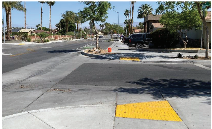
(New ADA-curb ramps at Catalina Way and San Pablo Avenue. Source: Palm Desert Safe Routes for Older Adults Walk Audit)
