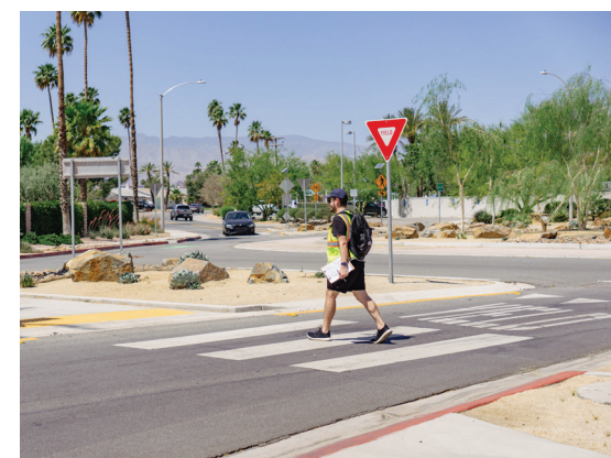
High visibility crosswalks, pedestrian refuge islands, Class III bicycle sharrows, and a roundabout were recently installed at California Drive/Michigan Drive and Avenue of the States.
