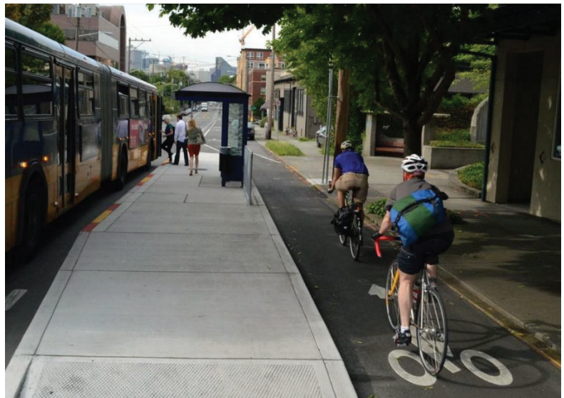
(A bus bulb with cut-throughs for a curbside bike lane. Source: nacto.org)
