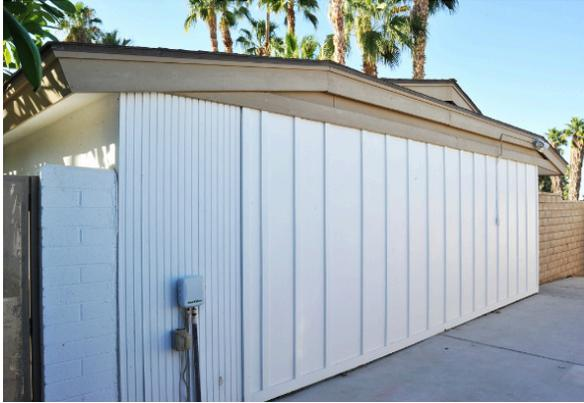
**Figure 18** - Existing east facade wall after removal of roof overhang
