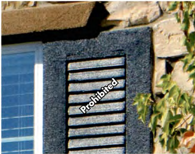
Example of prohibited embedded shutter
