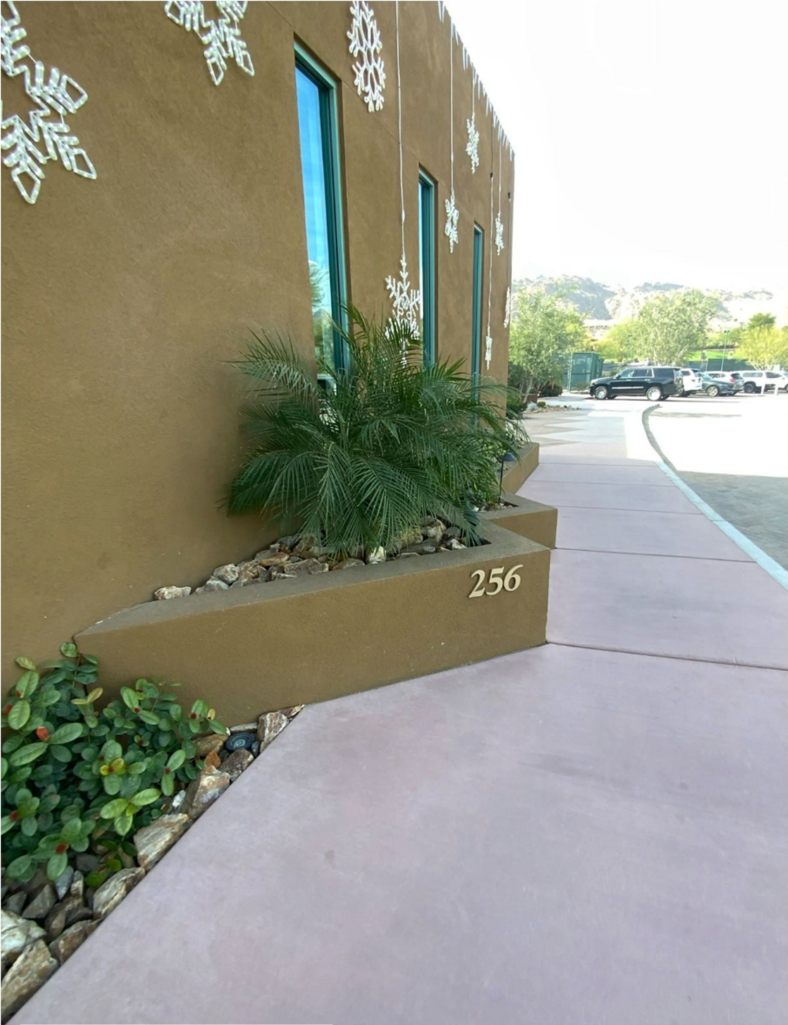
Existing north facade of fitness/weight room.
