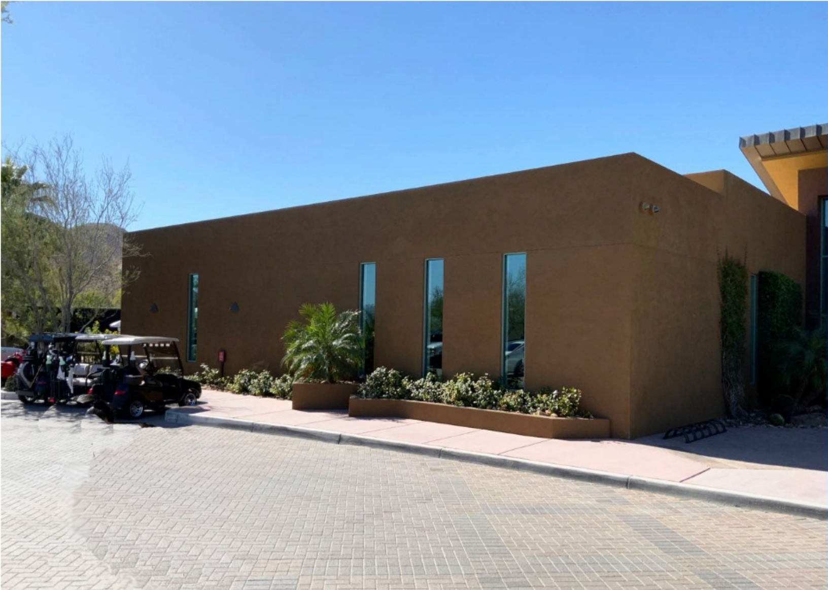
Existing east side of Spa - looking at existing fitness/weight room
