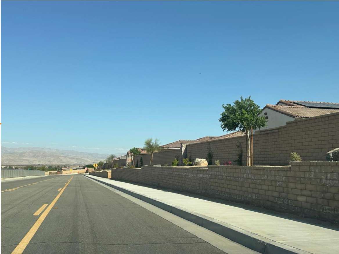
Perimeter Retaining Wall on Dolce Avenue moving east towards Cortesia Way
