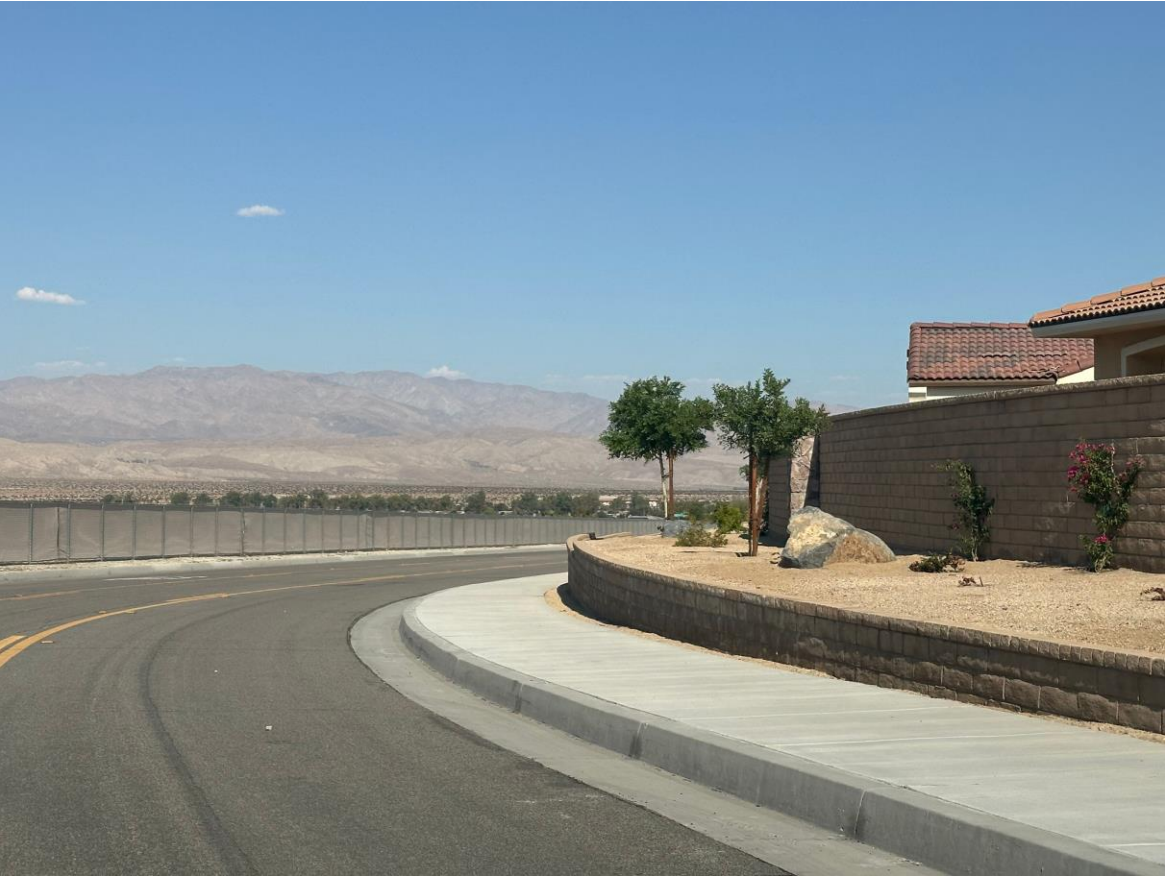
Perimeter Retaining Wall on Dolce Avenue near Gateway Drive looking east
