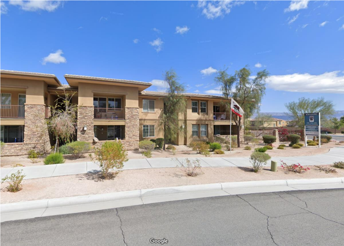
The Enclave at Gerald Ford Drive and Gateway Drive looking south
