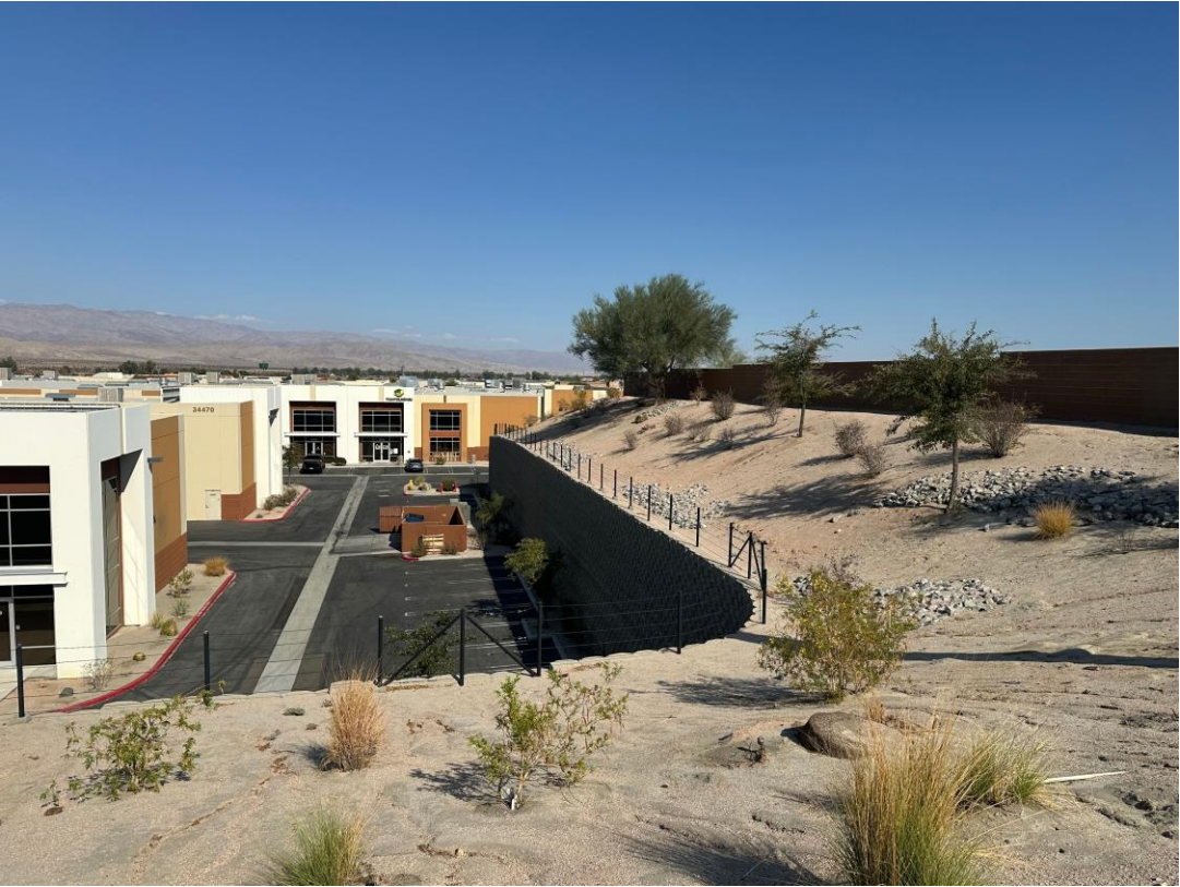
Pads below street retaining walls – Gateway Drive Looking northeast towards existing business park
