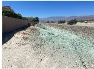
Chemical Dust Suppressant (CDS) Application: Soil binder is routinely applied to inactive or high sensitivity areas to control dust emissions. See attached records.
