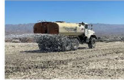
Active Site Watering – High-capacity water pulls and trucks are actively treating unpaved roads and active earthwork areas.
