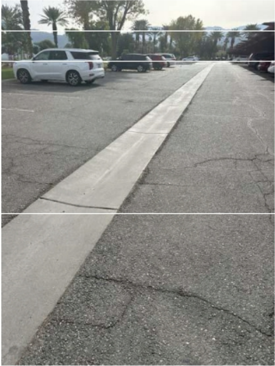
The area sheet flows to V-ditch areas to a Catch Basin. No drainage issues are found.
