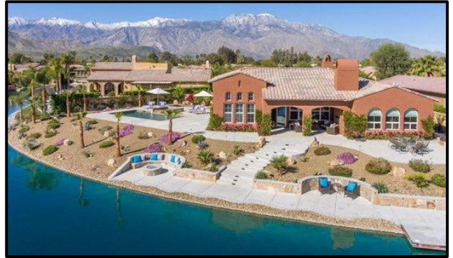
Pool & spa construction, new dock, deck, fire pit, and BBQ area (Rancho Mirage, CA)
