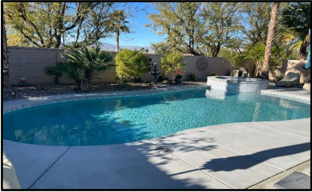
33' x 14' freeform pool & spa construction (Indio, CA)
