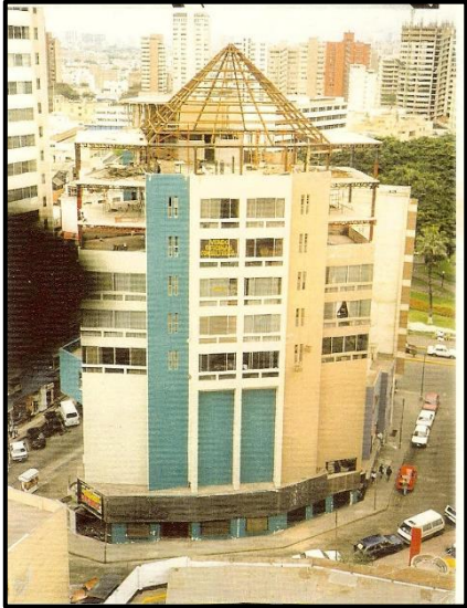
La Piramide Sky Room during construction (Lima, Peru)
