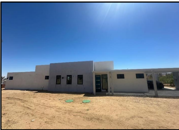
New single-family residence construction (Joshua Tree, CA)
