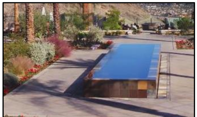
Water fountain construction for The Ritz-Carlton (Rancho Mirage, CA)
