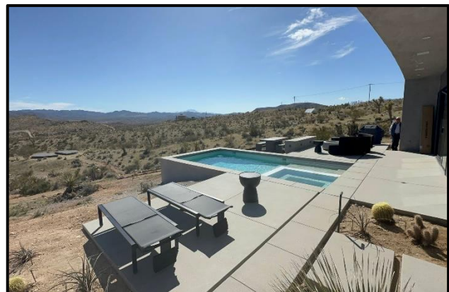
24' x 12' pool & spa construction (Yucca Valley, CA)
