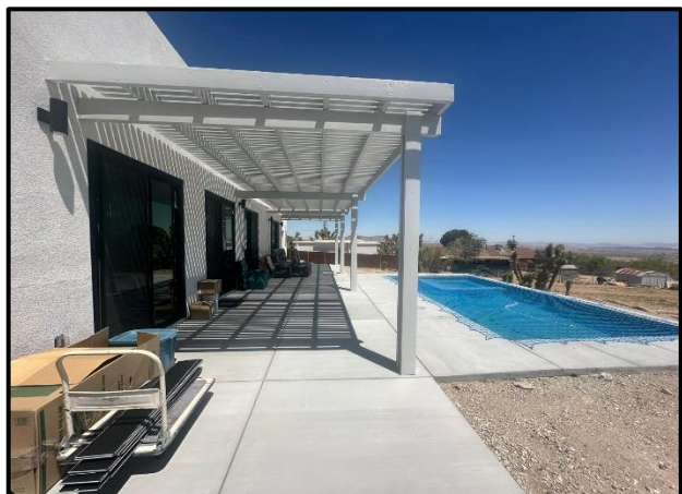
24' x 12' pool & spa construction for new single-family residence (Joshua Tree, CA)
