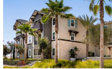
▲ This multifamily project uses multiple building materials through various transition techniques. Materials change at the inside corner of two building planes intersecting and a belt course horizontally divides the building and changes material. See ODS 4.5.2(a) and 4.5.2(c).
