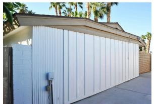
Figure 18 - Existing east facade wall after removal of roof overhang
