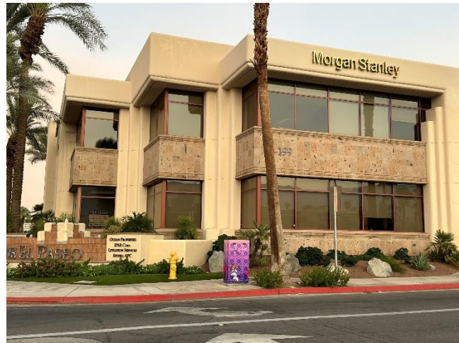
Two-story building within the D-O, Downtown Core Overlay district.
