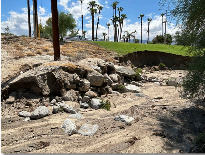
Looking South: SCE Power Pole
