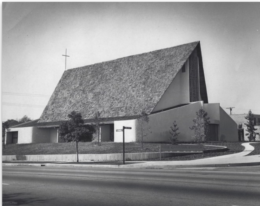
Figure 14. The First Christian Church in Pasadena, designed in 1966 by Galbraith, showing his shift towards the Late Modern hybrid. Photo from Irenic Projects.
